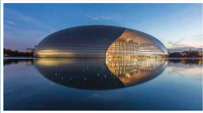
Beijing National Centre for the Performing Arts ,China
