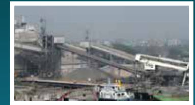
Meghna 2 Narayanganj, Dhaka
